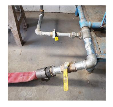
In March, the Meter department made improvements to the meter test bench; reducing test times from an hour to 15 minutes. Dustin Mills and Derrick McMichael came up with an idea to fix the current water tank drainage problem. They cut the pipe and installed a ball valve; making it possible to drain the water more quickly through a hose. They also mounted a shelf for added organization. These improvements will help the meter department test 3/4" to 2" meters more efficiently.
