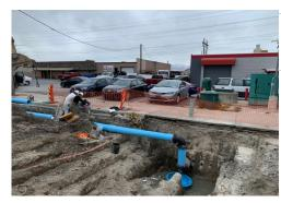
10-inch bypass piping near existing wastewater pump station
