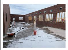
Building Addition -Completion of masonry work for the addition
