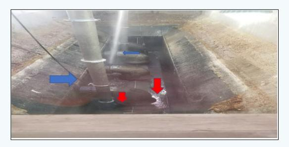
This shows the vactor tube (blue arrows) pulling grit from the bottom of the wet well. You can see on the sides of the pump suction tubes the grit on the bottom of the wet well floor (red arrows).
