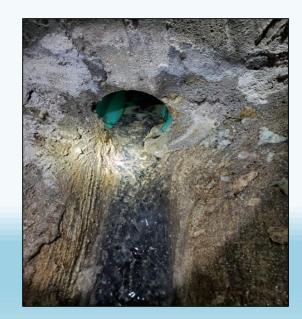
Depicts concrete in a lateral that comes into a manhole, which caused a home to backup, mainly because wipes were being used. Concrete was removed.
