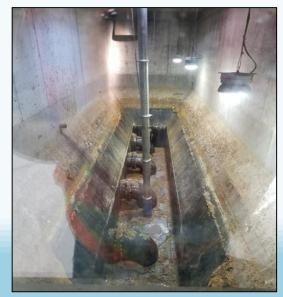
This is a picture of the wet well with the "grease blanket" before the cleaning begins.
