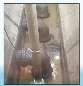
Here we have taken the water down to the level below the suction of the pumps, and to the level of the grit.
