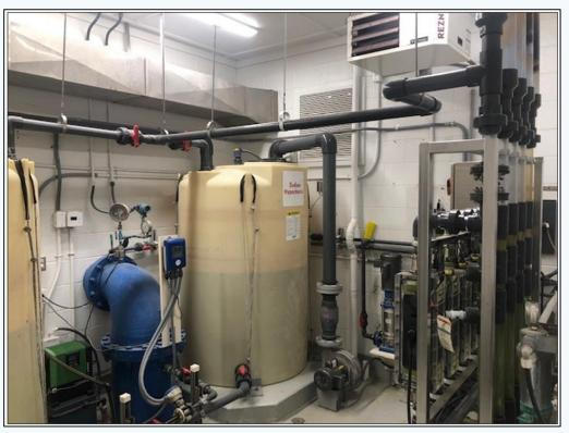
The picture above is the inside view of the sodium hypochlorite room at Well 8. The large tanks to the left of the picture are the storage tanks for the sodium hypochlorite solution that we use to disinfect our water. To the right of the picture is a side view of the new PSI sodium hypochlorite generation system. The new system was installed and put into operation in July of 2020.
