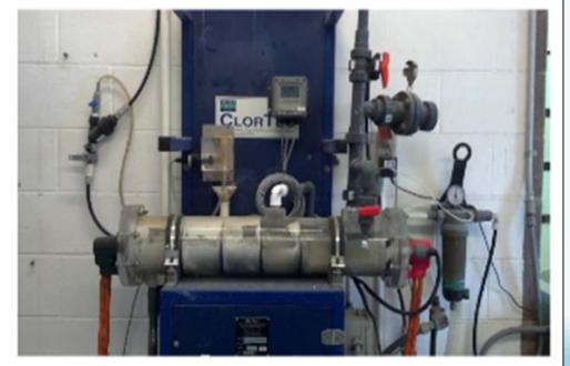
The picture above is the old sodium hypochlorite generation system that was replaced with the new PSI system at Well 8 in 2020.
