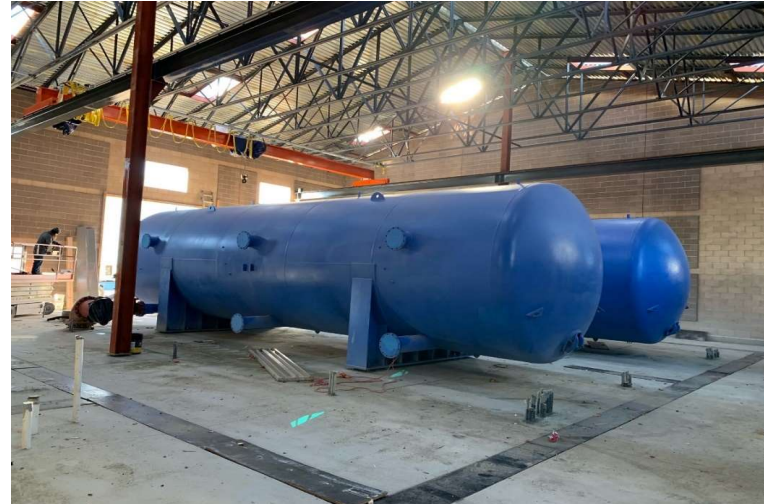
Roof and crane installation
