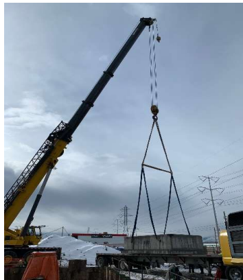
Crane lifting precast pig launch vault base from truck
