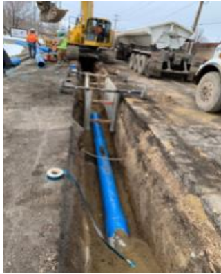
12-inch PVC installation along 4700 South
