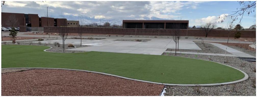
Finished concrete pad for demonstration garden area
