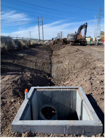
Excavation for detention pond. Installed catch basin
