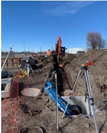
15" Storm Drain Installation
