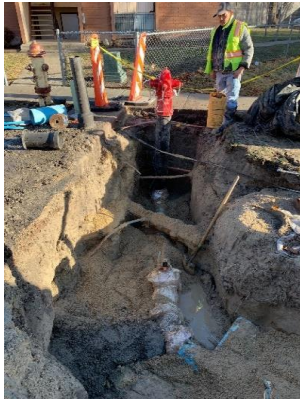
Fire Hydrant Installation
