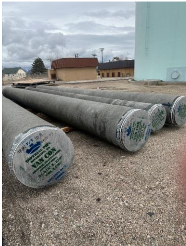
30" and 24" stockpiled pipe on site
