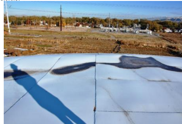
Acord Reservoir Roof
