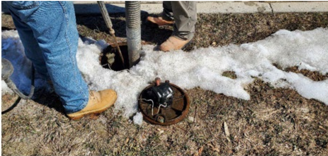
Water crew identifying water line material.
