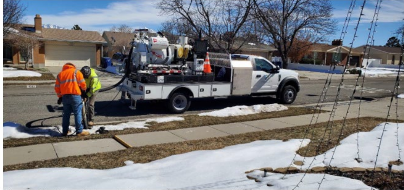
Water crew identifying water line material using a valve maintenance vehicle.
