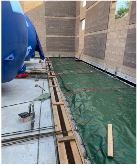
Concrete Flatwork Preparation
