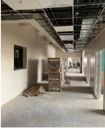
Ceiling light installation
