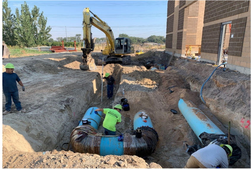
Water Pipe Installation
