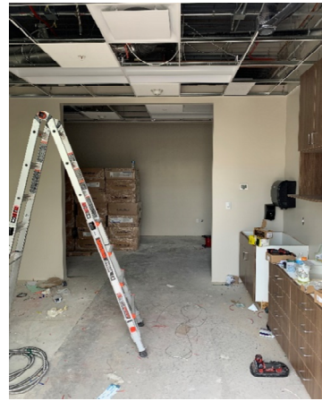
Break room cabinets
