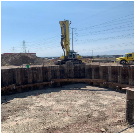
Excavation by means of sheet piles
